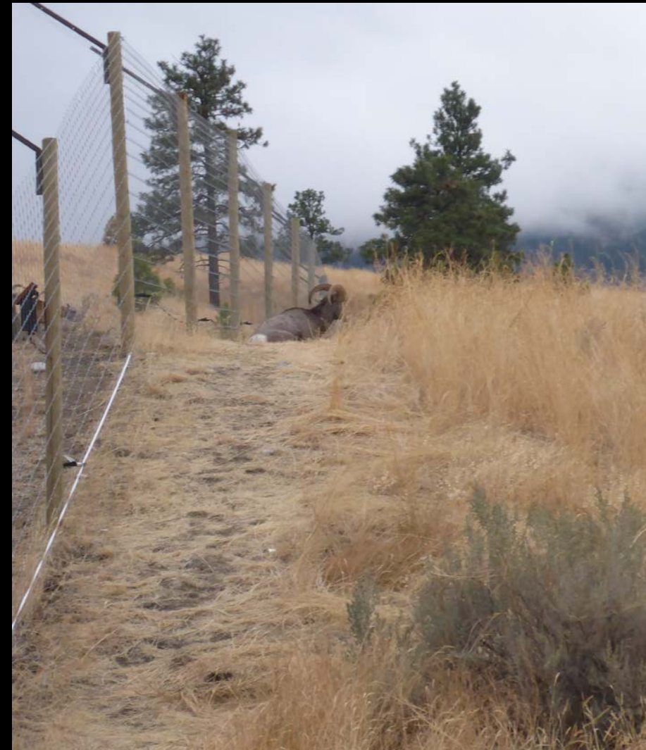
2.4m woven wire with electric outrigger overhang at 45 degrees (double fence to prevent nose-to-nose)
